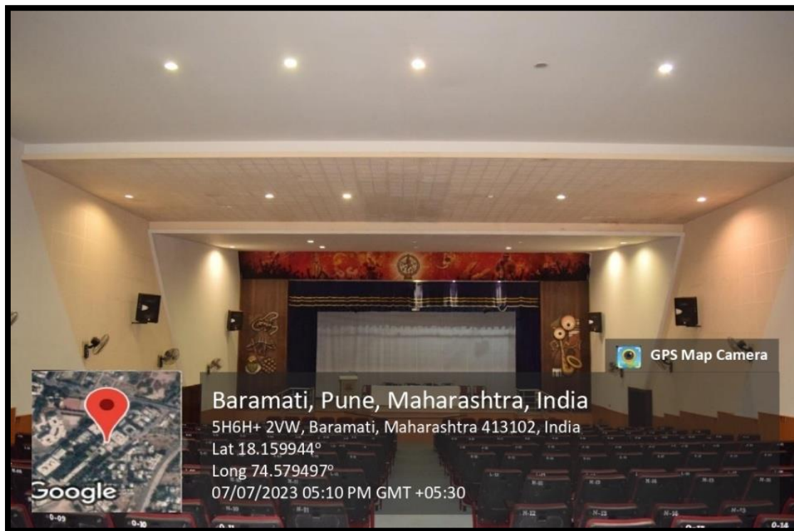
LED lights installed in Auditorum of College- Jivraj Hall
