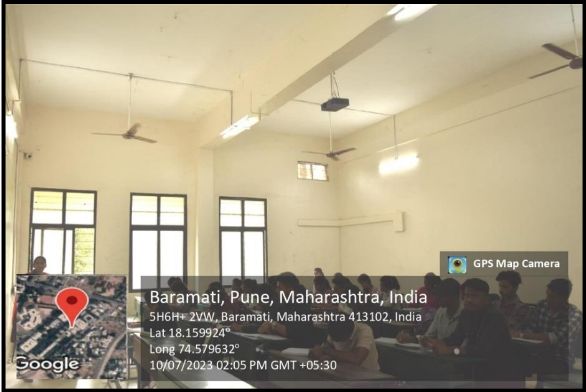
LED lights in Classrooms
