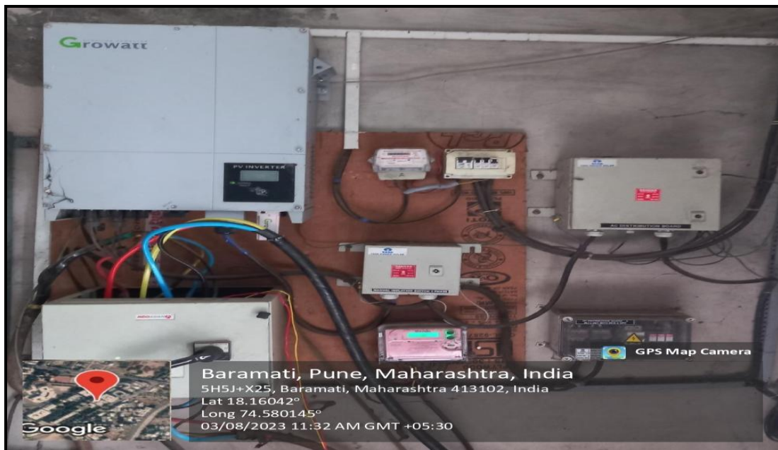
Setup of Wheeling to the Grid
