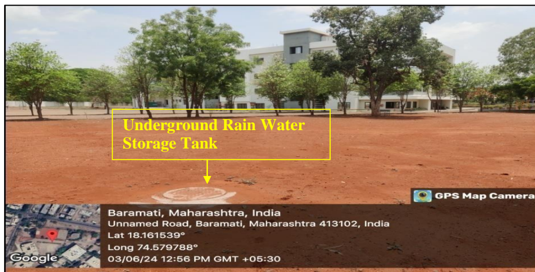
Play Ground Area: Rain Water Harvesting System
