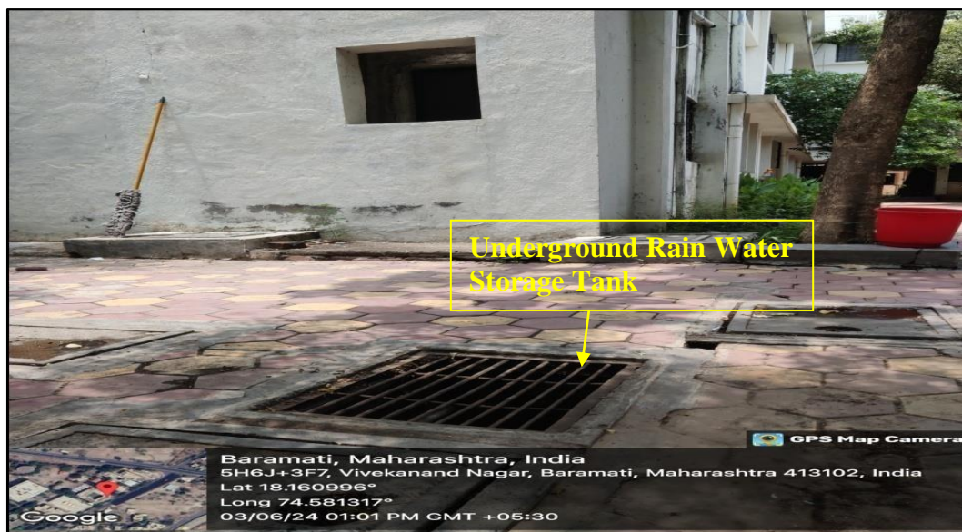
Near Girl's Hostel: Rain Water Harvesting System
