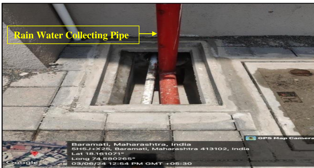
Physics-Micro Department: Rain Water Harvesting System
