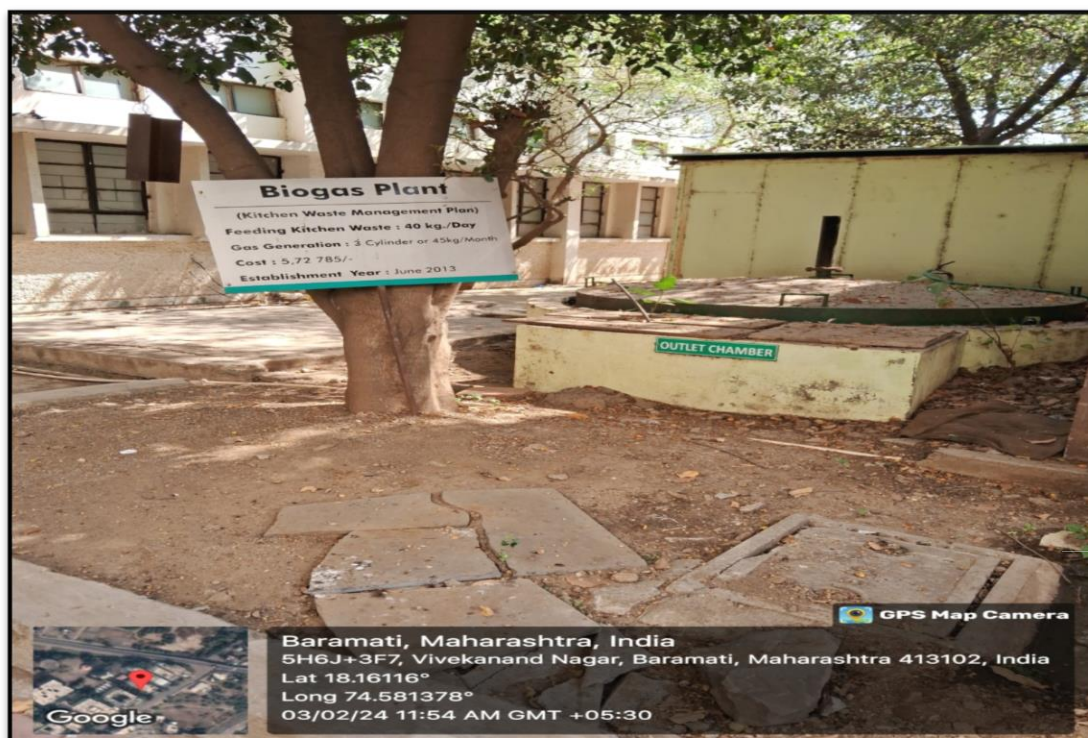
Biogas Plant for biodegradable waste
