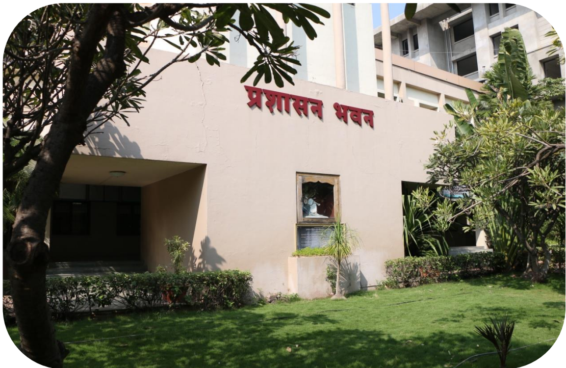
Lawn in front of Administrative Building
